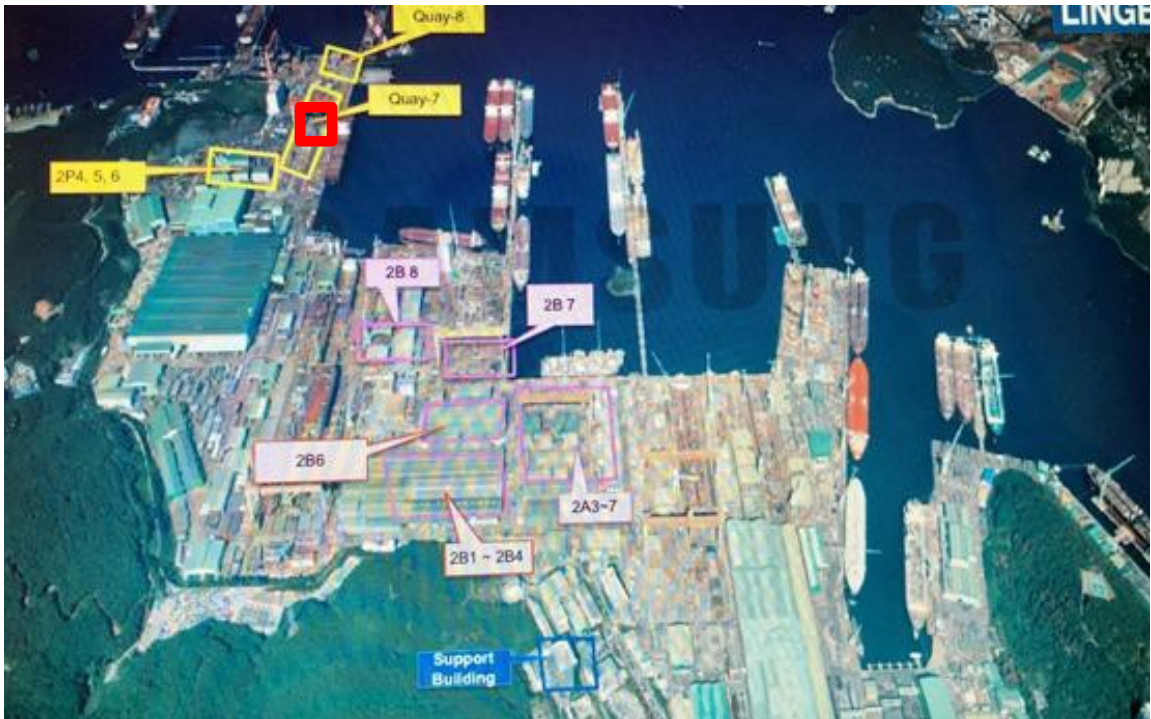
Overview of the SHI Yard. Construction of the Martin Linge module took place on Quay 7. The red square indicates the approximate location of the area dedicated to the construction of the Martin Linge topsides (illustration provided by TEPN).
